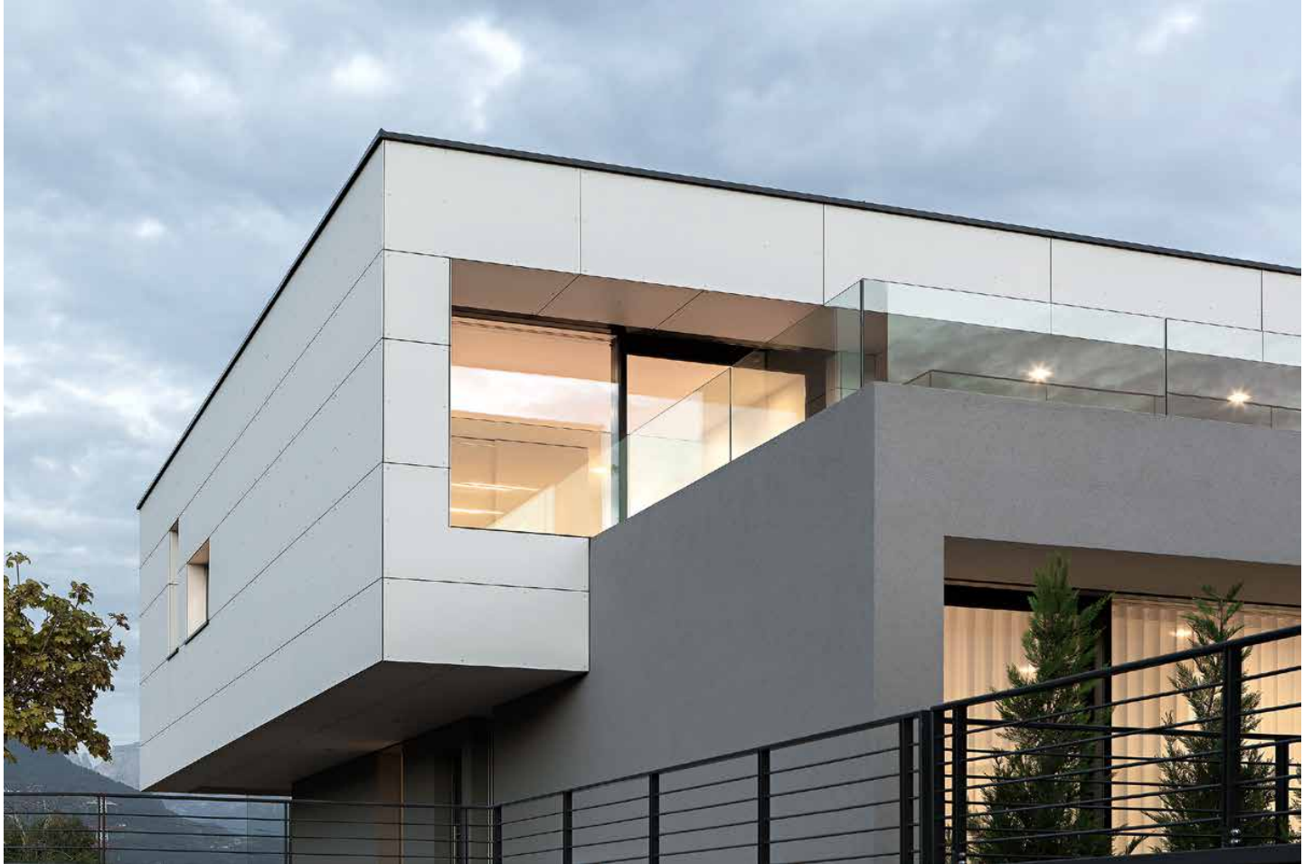
A change in cladding material from light grey plaster to white Swisspearl panels accentuates the two separate units of the building.
